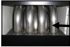
Heat Exchanger tubes located behind grill
